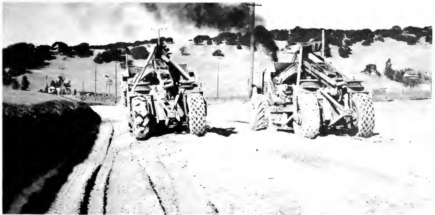
Carryalls engaged in grading on Vallejo-Napa highway between Napa Wye and Vallejo. Paving on this stretch is now nearing completion.
